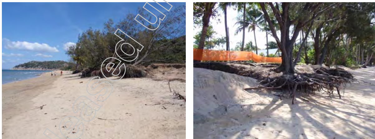
Figure 1-3 Beach erosion on Nelly Bay Beach
