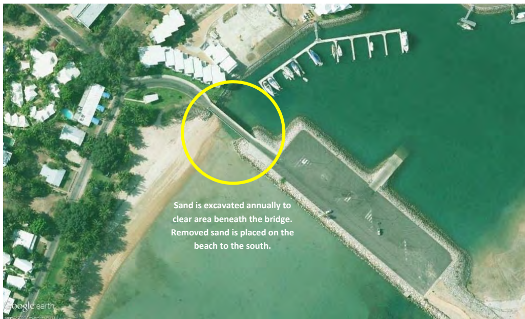
(b) Sand cleared from beneath bridge to allow tidal flow
