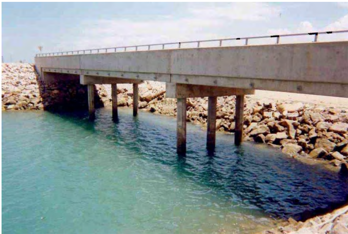
Figure 4-2 Bund preventing tidal flow beneath bridge (circa 2002)
