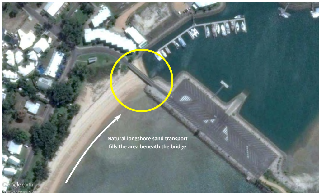
(a) Sand blocking tidal flow beneath bridge
