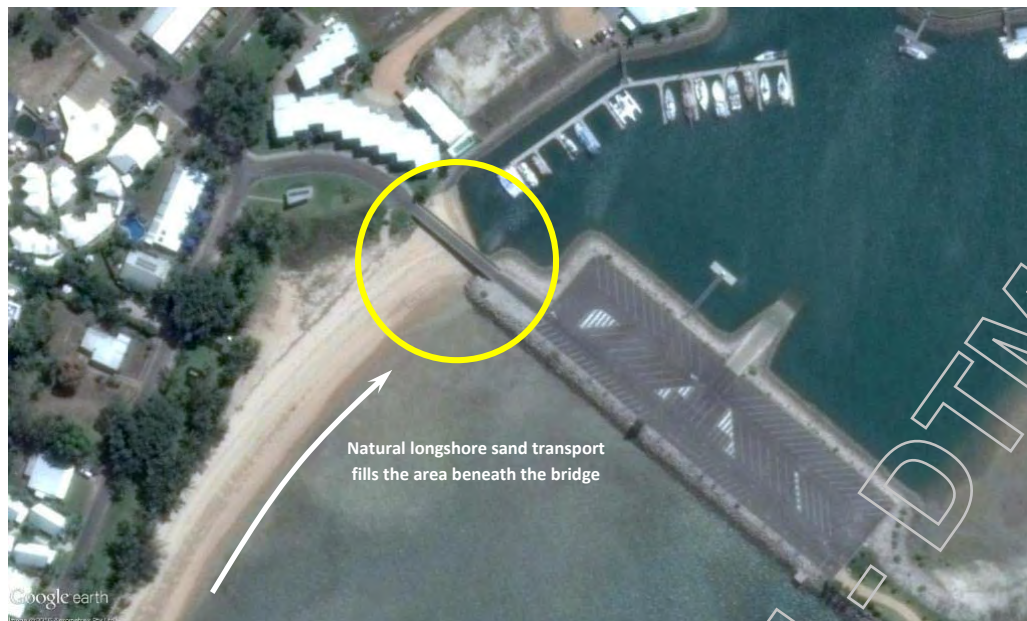
(a) Sand blocking tidal flow beneath bridge
