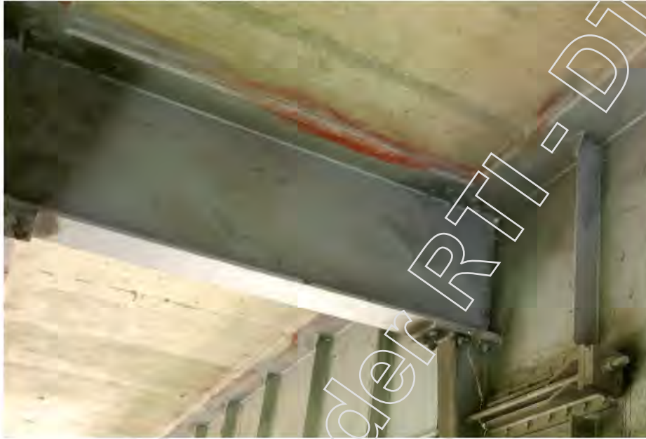
Figure 40: Typical internal cross girder member and connection.
