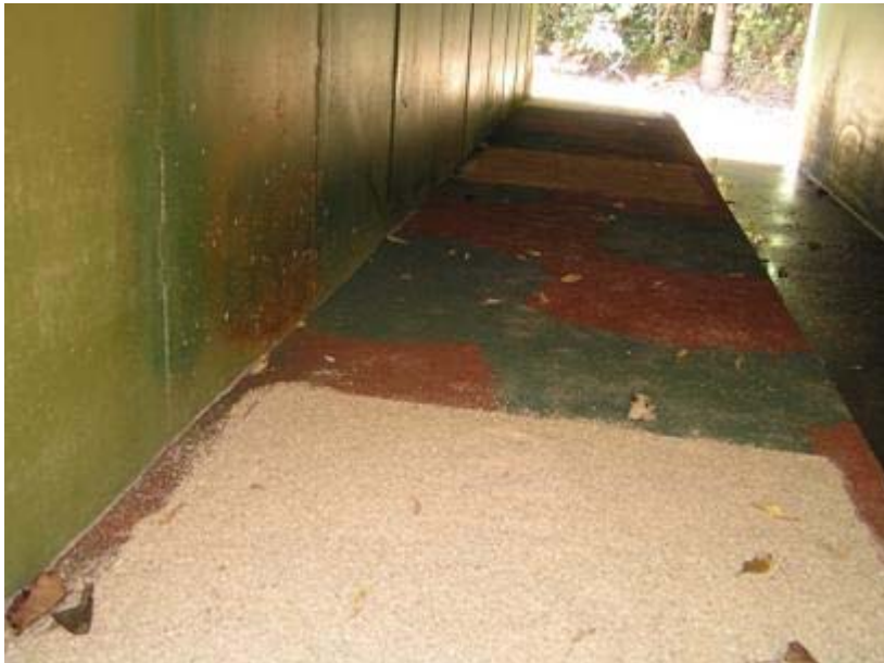
Figure 4.2.7 Underpass with two sand plots used to monitor fauna use.
