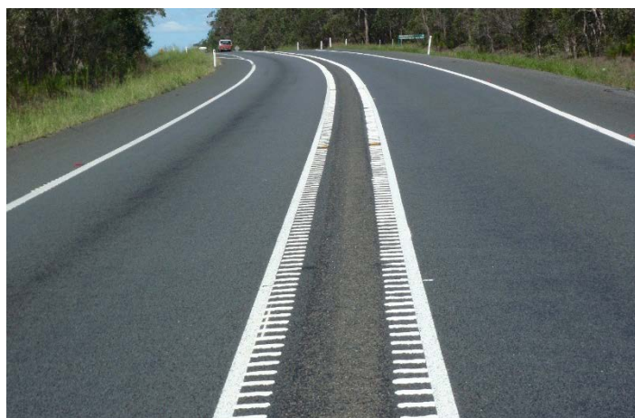
Figure 2 Wide Centre Line Treatment with Audio Tactile Line Marking
