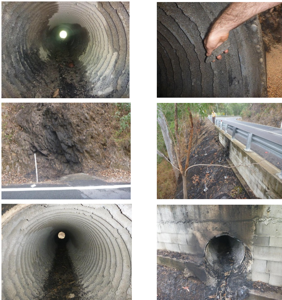
Figure 1.2 – Vandalised pipes
