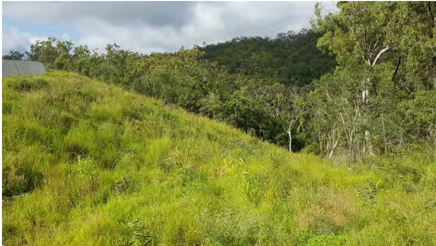
Figure 5: Successful organic blanket treatment on road batter
