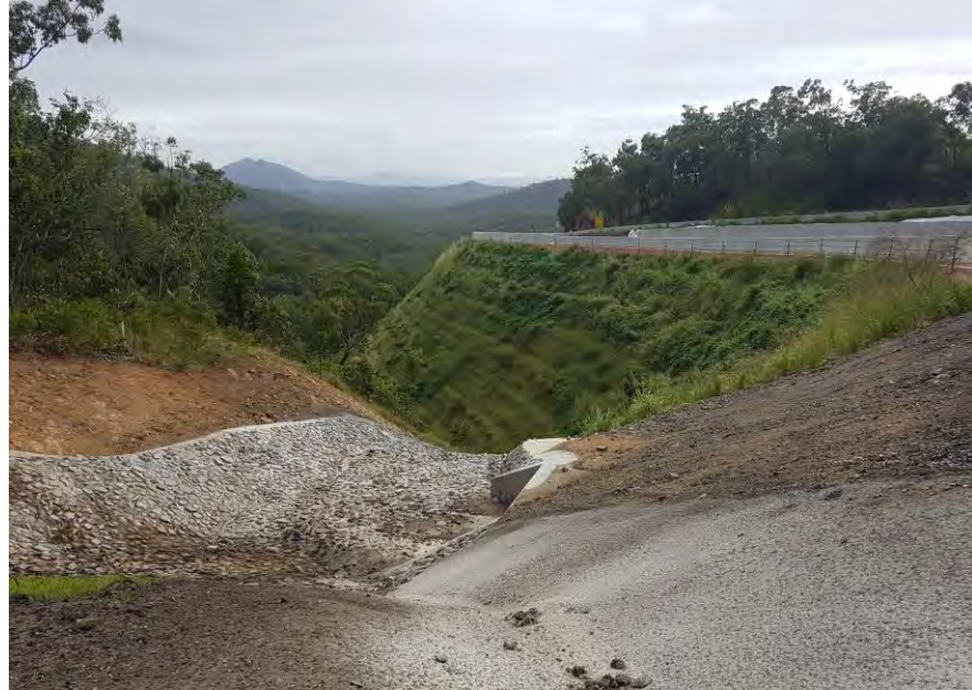
Figure 10: Looking at landscaped REE from Culvert 6C
