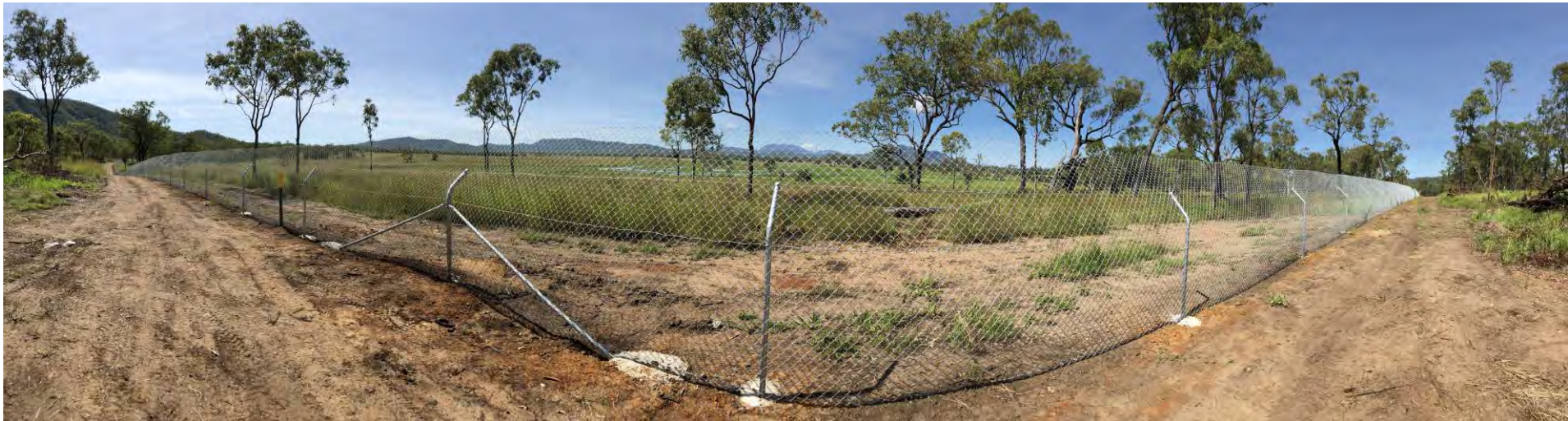
Figure 15: Fauna exclusion fencing at Denison Creek constructed in compliance with 2015/7552 Condition 11.
