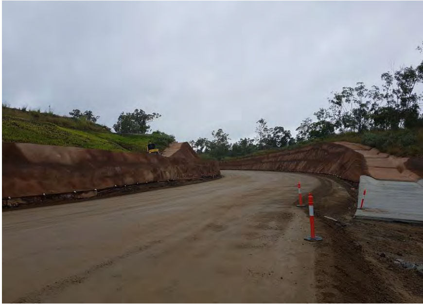
Figure 9: Pavement works at Cut 107
