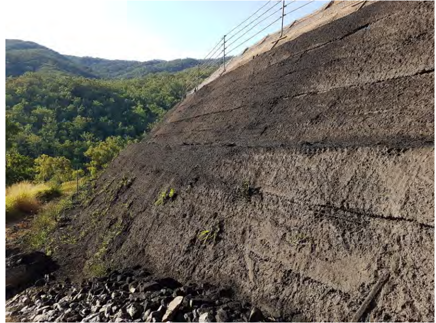
Figure 8: Application of organic blanket at a REE
