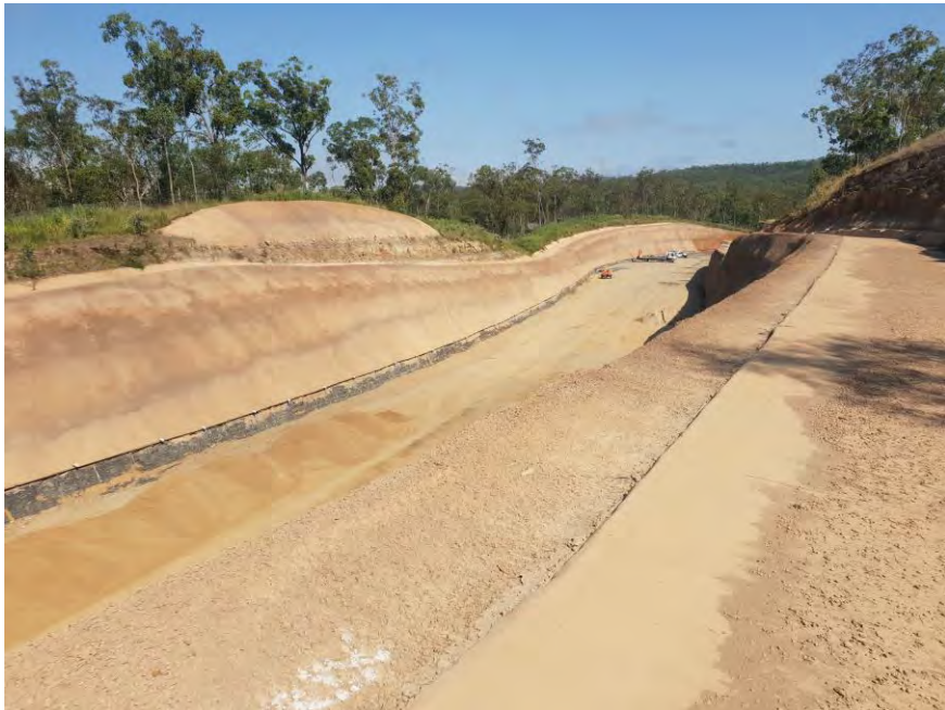
Figure 7: Completed shocrete and CTB correction at Cut 107
