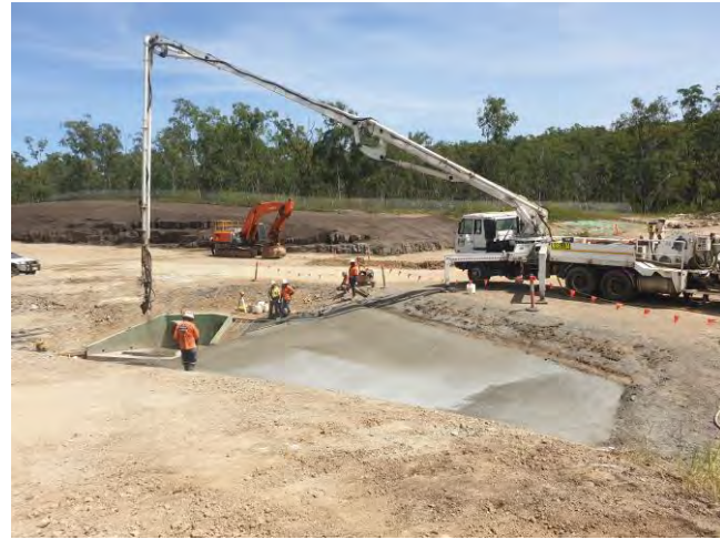
Figure 6: Concrete works at Culvert 6A.
