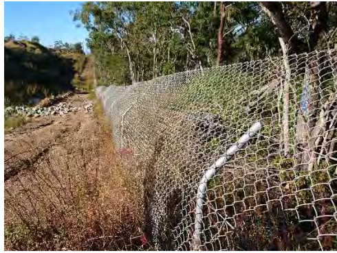
Figure 19. Koala barrier fencing erected in association with the upgraded Eton Range upgrade of the Peak Downs Highway.
