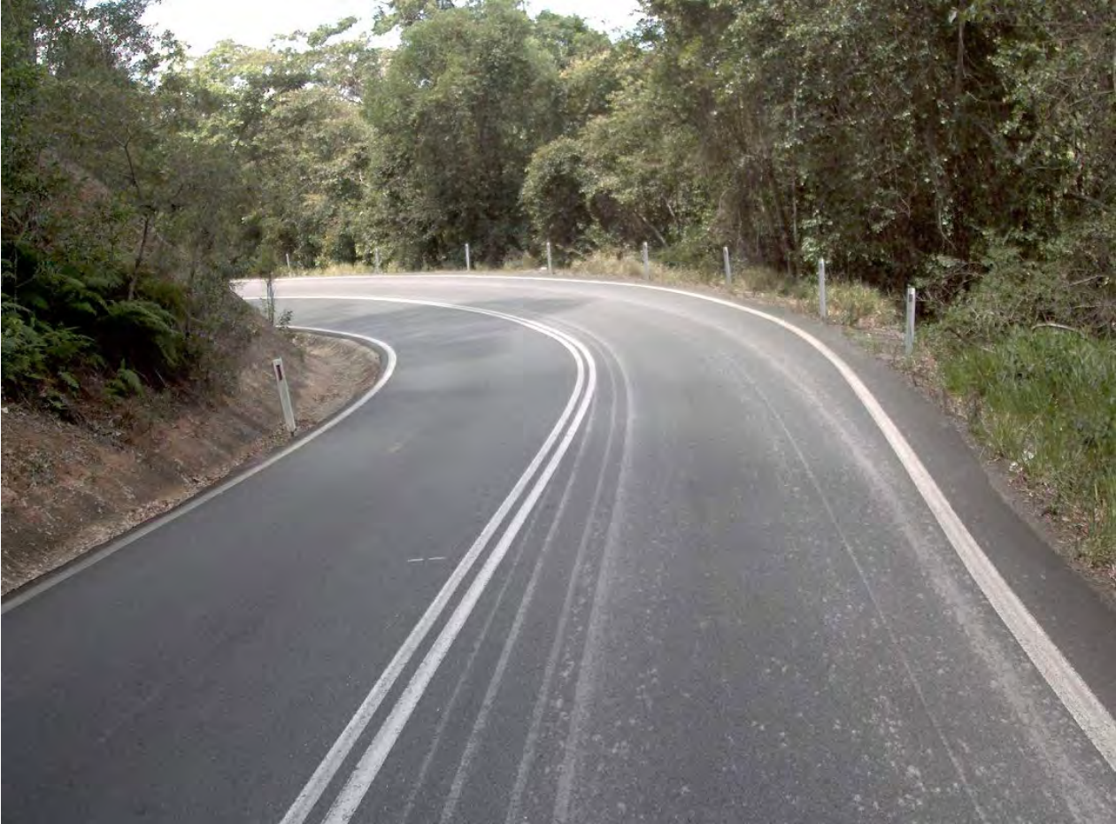
Figure 23: Photo showing location of crash involving a heavy vehicle on Kin Kin Road
