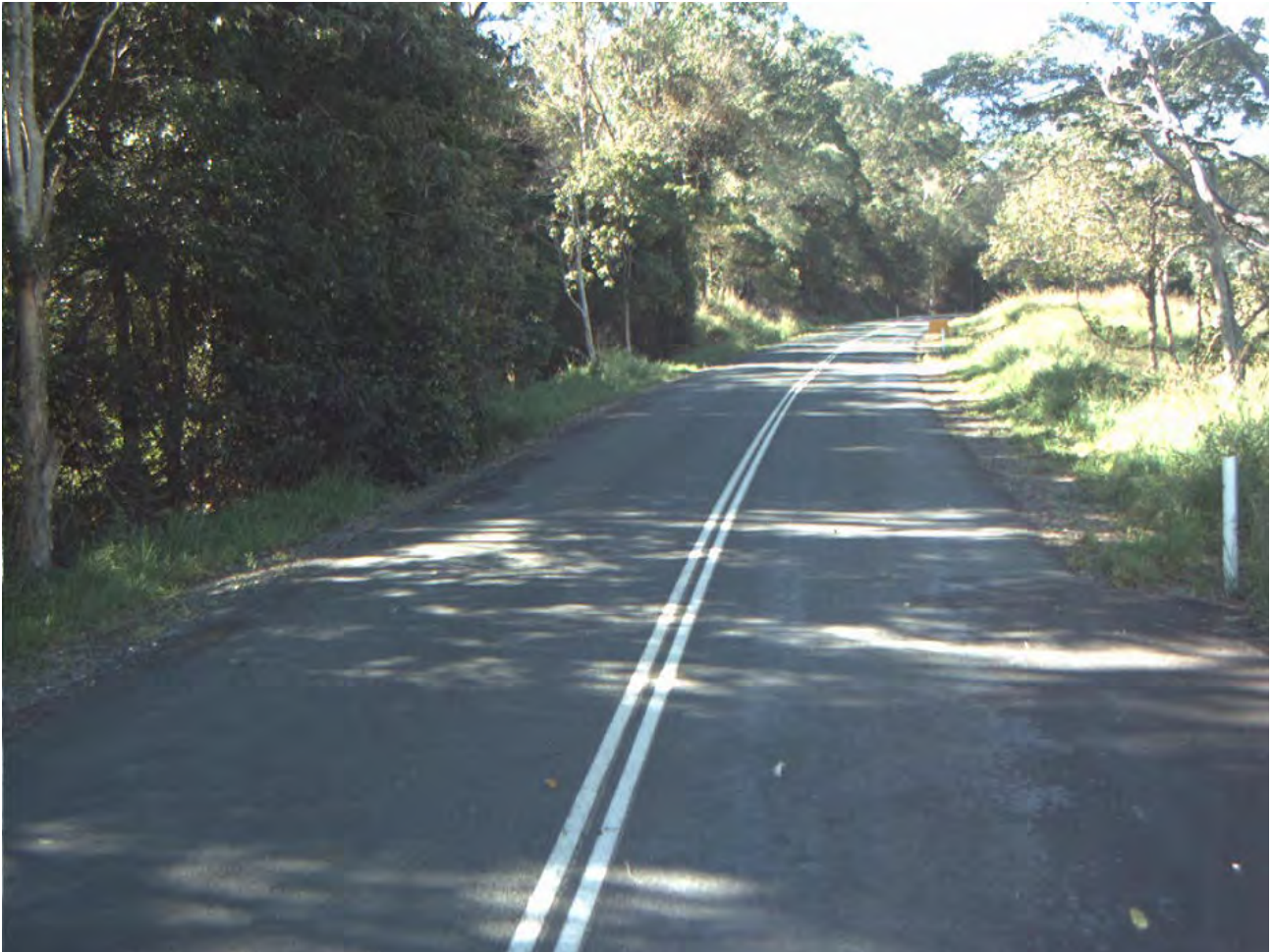
Figure 22: Photo showing location of fatality on Kin Kin Road
